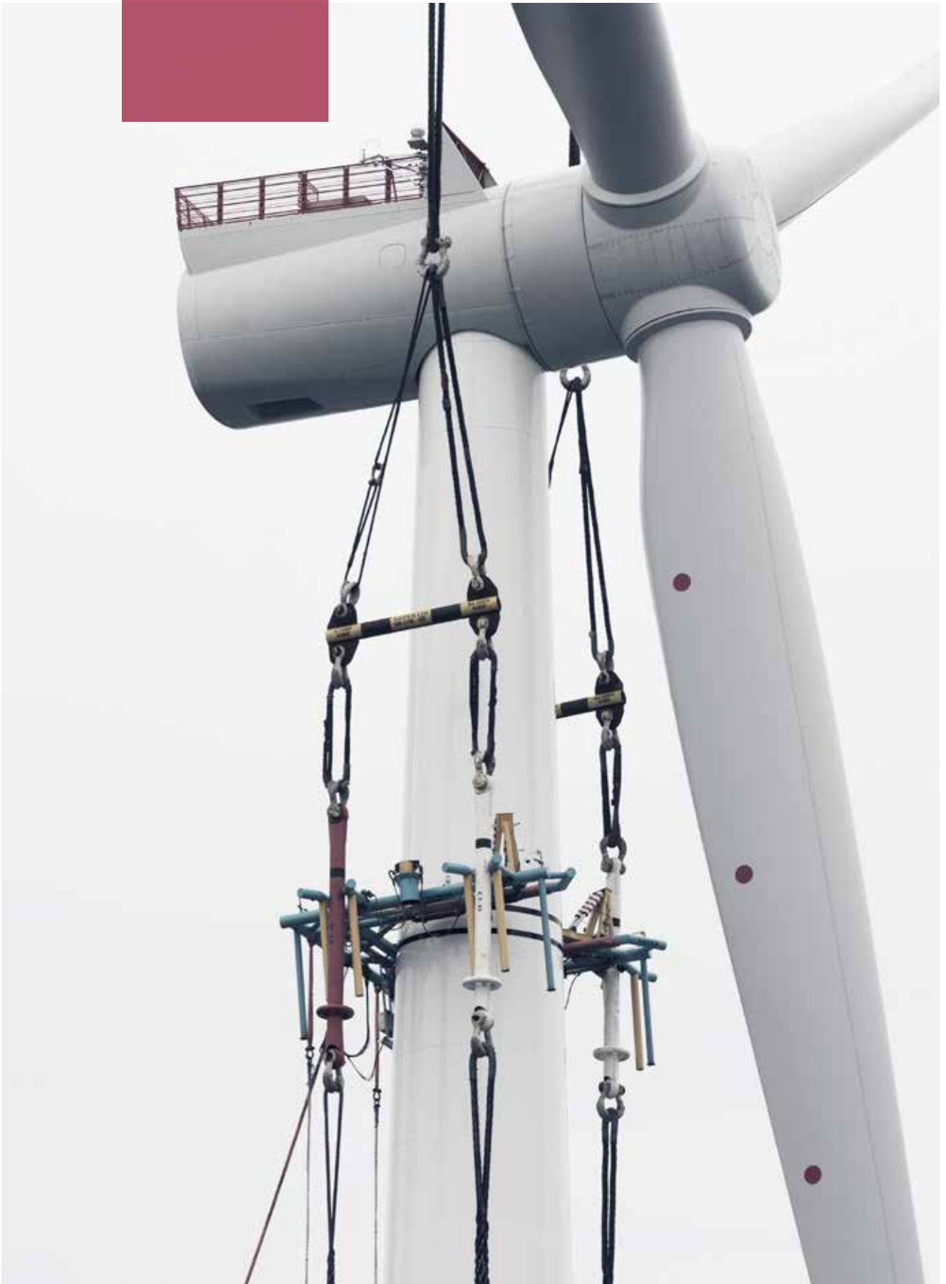
Statoil - Hywind Scotland mating of first wind turbine. Photo: Kjetil Alsvik
