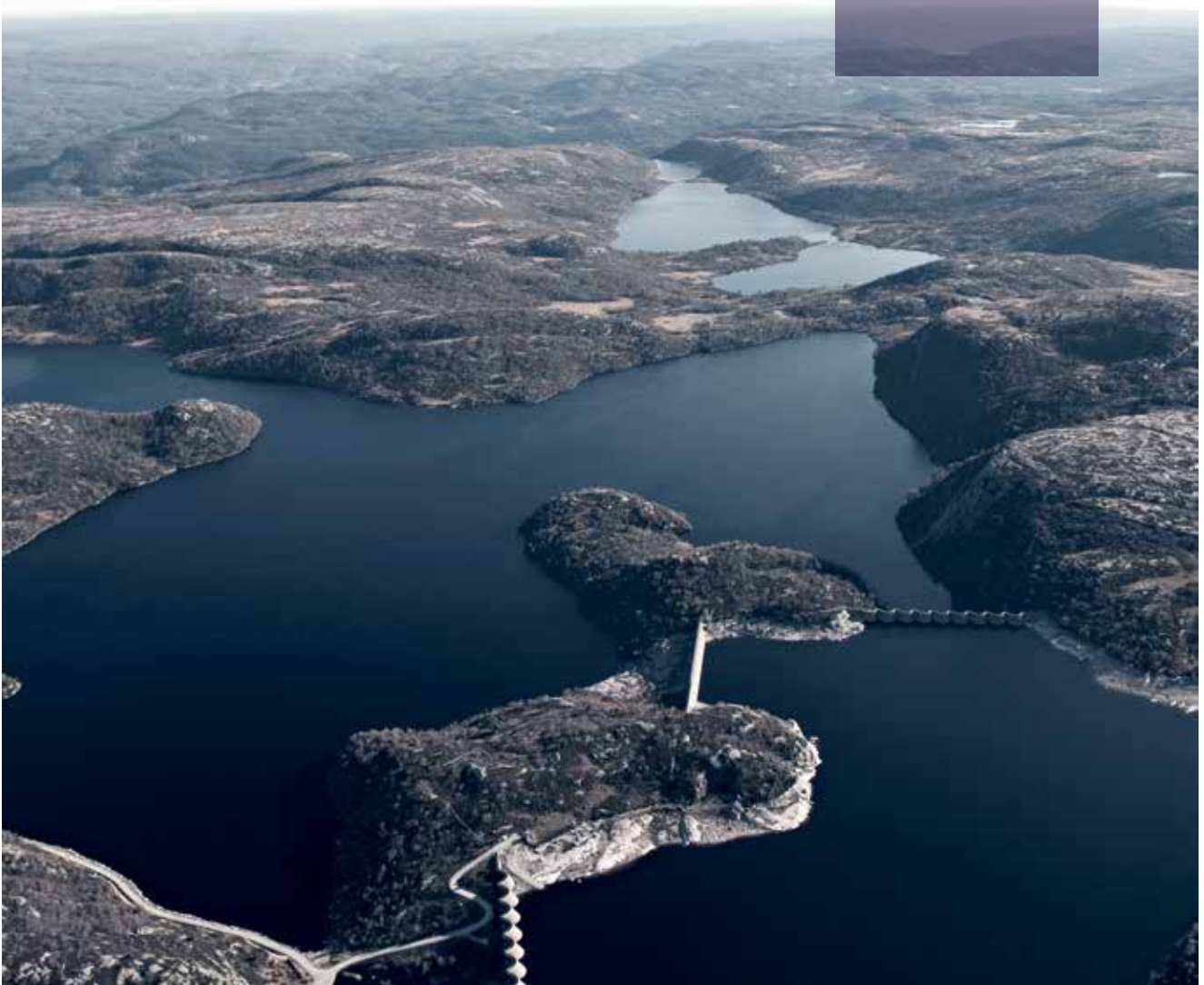
Skjerka hydropower plant. Photo: Agder Energi
