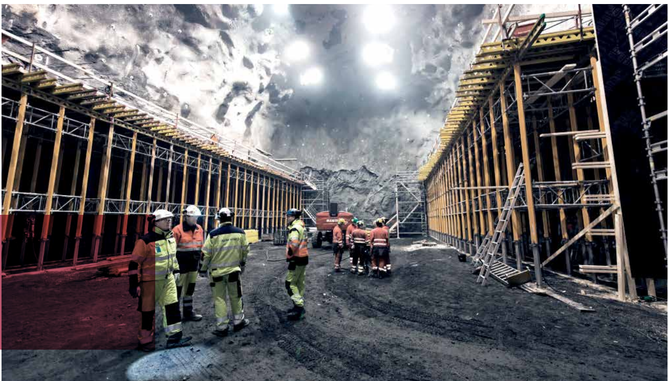
Power house under construction, Iveland hydropower plant. Photo: Agder Energi
