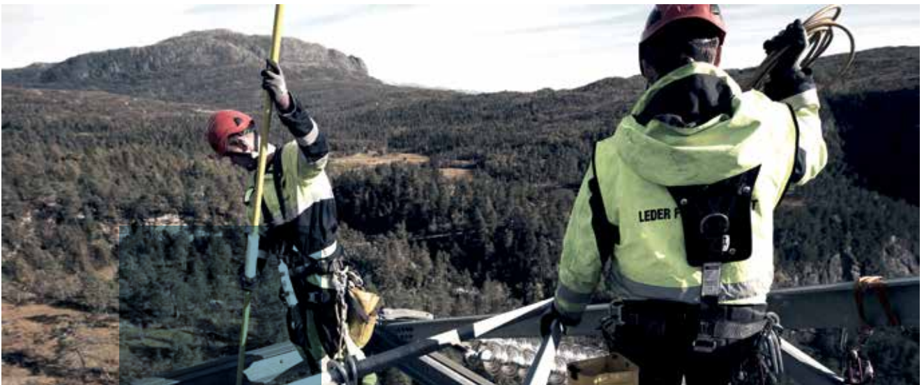
Transmission tower work, Statnett. Photo: Jahan Wildhagen
