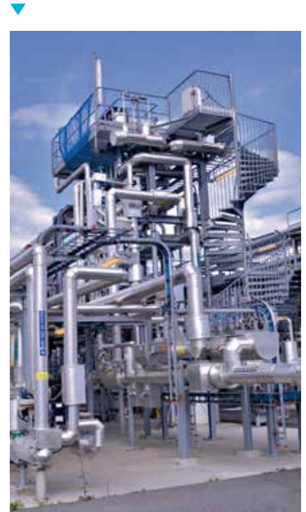
The Statoil test loop facilities i Porsgrunn. Photo: Anders J. Steensen
