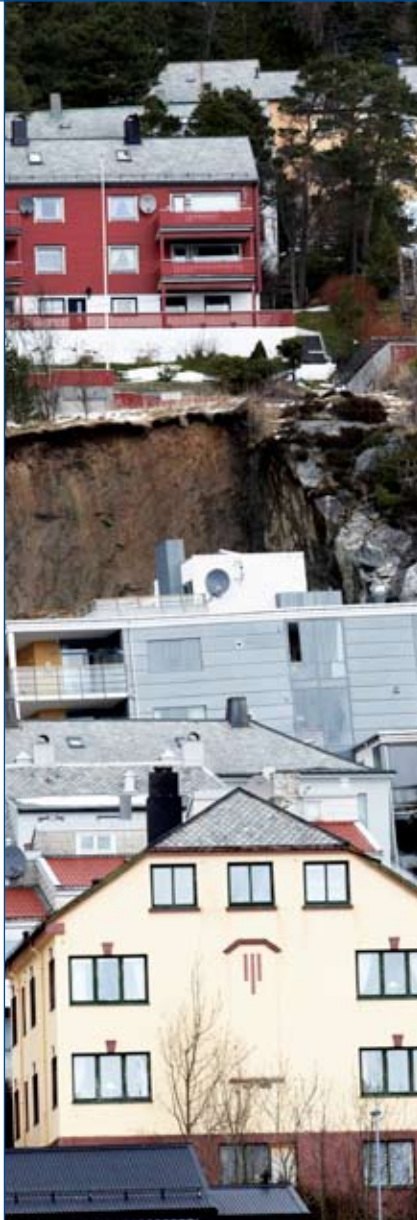
Five people died in Ålesund in March 2008, when a large boulder broke off the hillside and crushed the ground floor of an apartment building. Many Norwegian municipalities have not done enough to secure against rock slides. (Photo: Tore Kristiansen, Scanpix)
